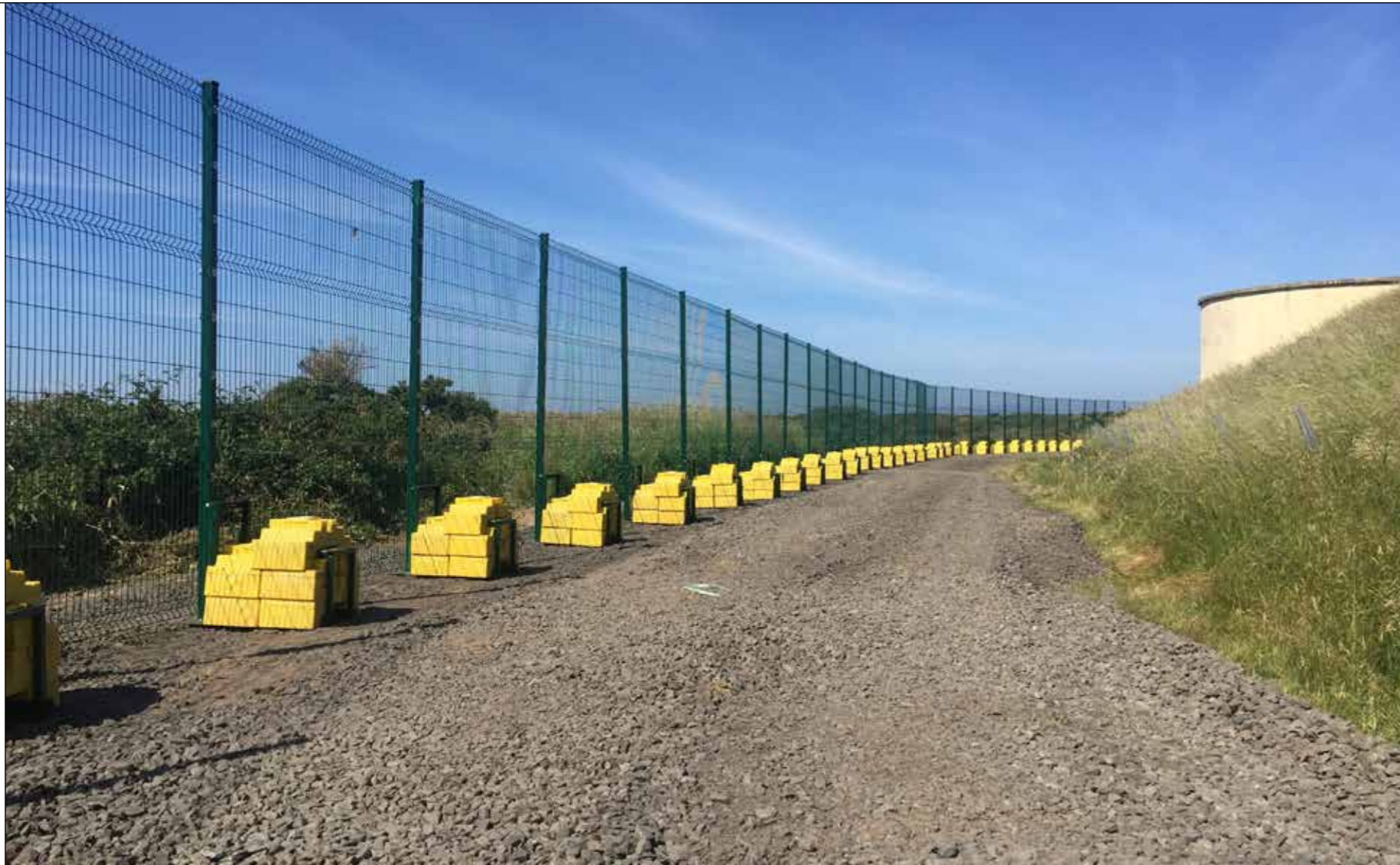
Above: Water-filled ballast options using tanks made from recycled plastic provide an environmentally friendly alternative to concrete
