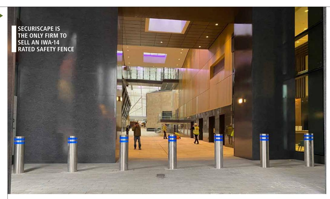
into the surface of a road or pathway. Depending on need, the bollards can either be immobile or they can be slid aside manually to allow a vehicle to gain access and pushed back into place to form an impregnable barrier.
