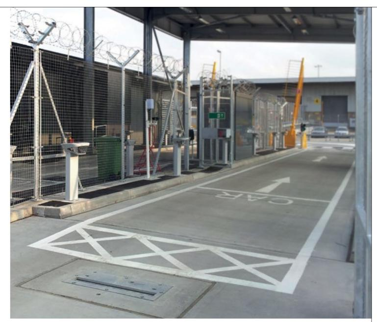
Gatwick has installed Chemring Technology Solutions' VehicleScan surveillance technology is that all vehicles can be checked and a complete view of the underside of those vehicles is presented for review. This gives the security team 100 percent coverage for the underside of every vehicle passing through the control gate.
